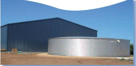
this application. Simply put, Aquamate knows this is not true. When a tank is full, the liner is pressed up against the inside wall, causing condensation to be trapped between the liner and the tank wall. The corrosion to ZINCALUME® steel is inevitable due to the moist conditions & the lack of oxygen (air), which ZINCALUME® steel requires to form its stable oxide films that would normally prevent further corrosion.
